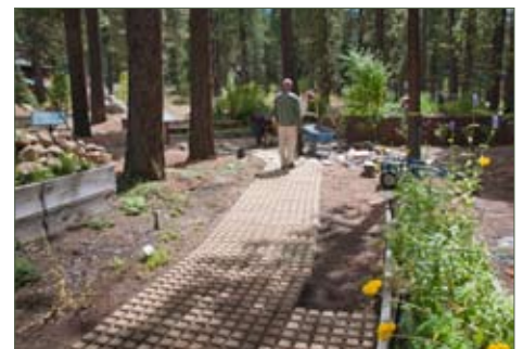
Installation of plantable walkway in 2010
