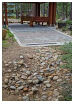
Driveway exhibit and infiltration basin
