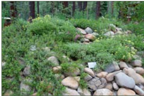
“Rip-rap” with vegetation
